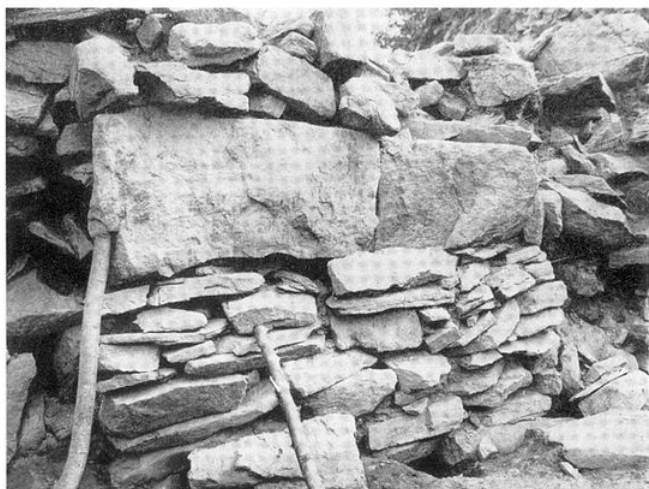
Inner bank with flat stone slabs immitating the so-called Cyclopean masonry.
