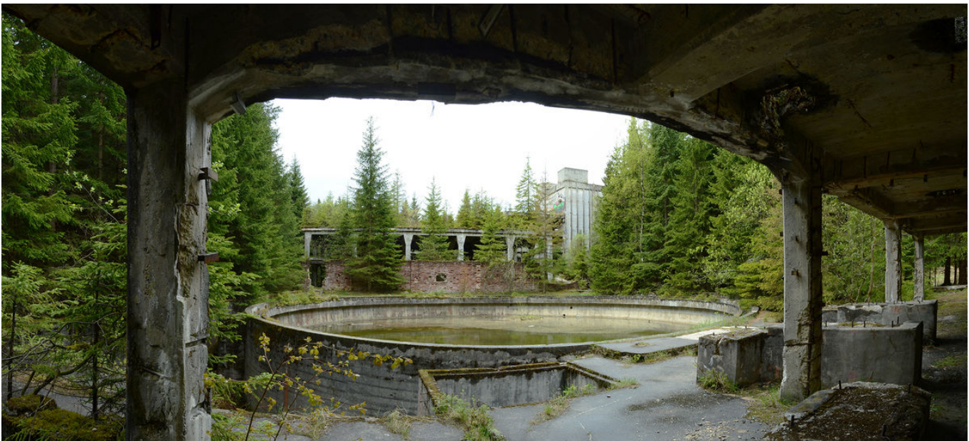
View across the originally roofed sludge condenser pond on the ore treatment plant with silos.
