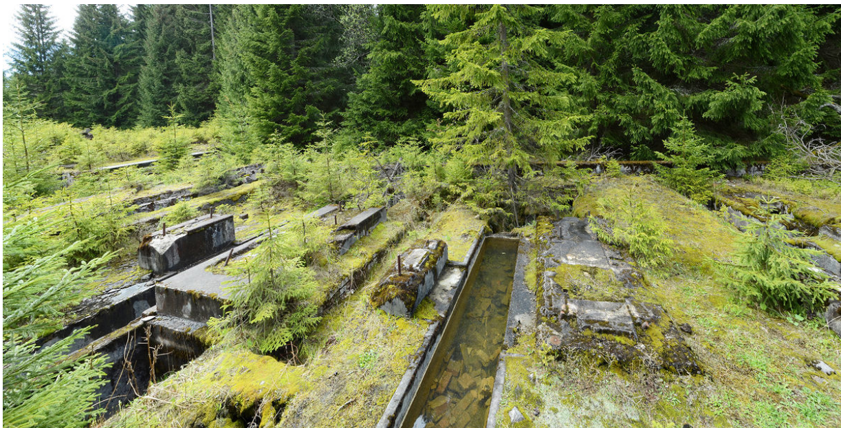
Concrete bases for mining devices and mine ventilation system.
