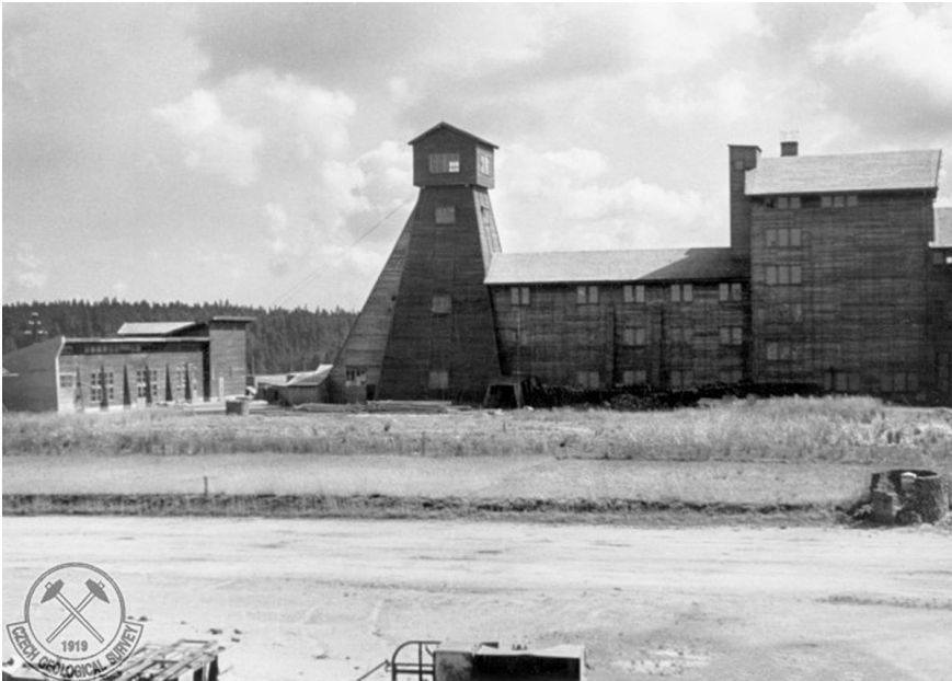
Historical picture of already dismantled mining tower (in the middle), engine house (left) and ore mill with ore silo (right).
