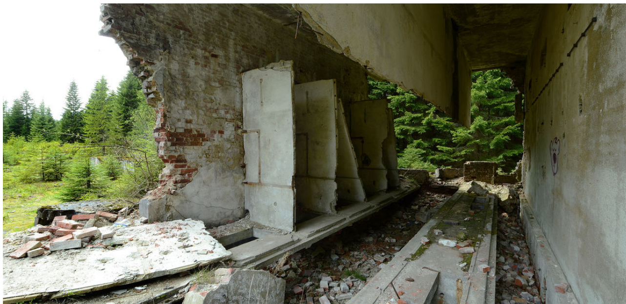
Former showers area.
