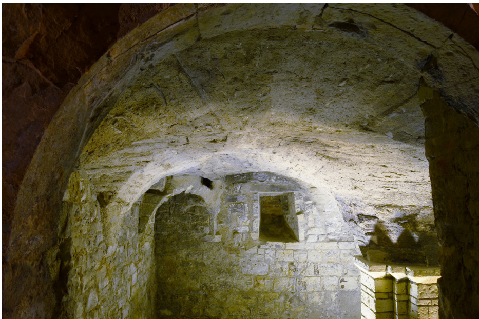
Southern chamber of the basement.
