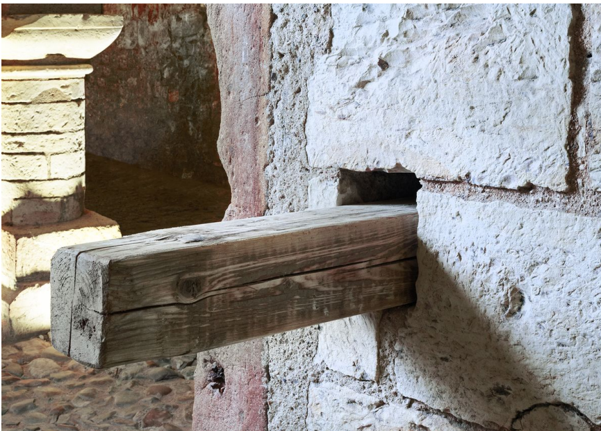
Bolt next to the entrance to the basement's southern room.
