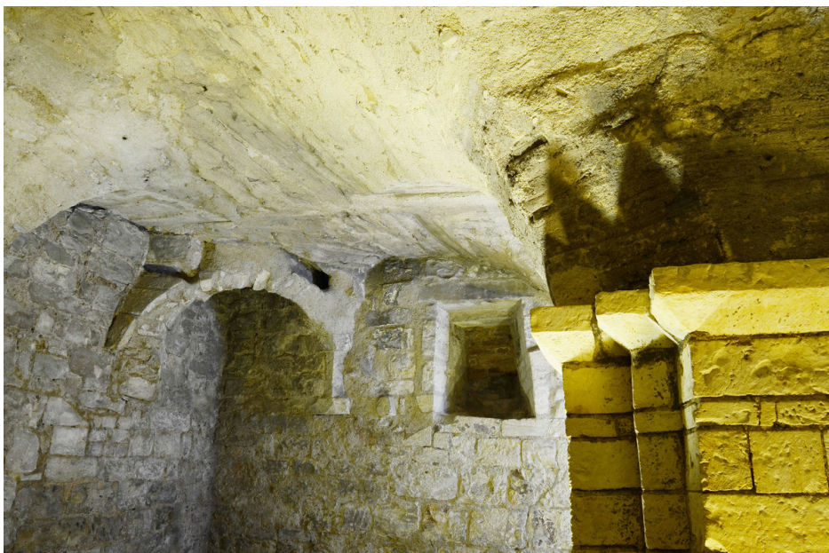
Southern chamber of the basement.
