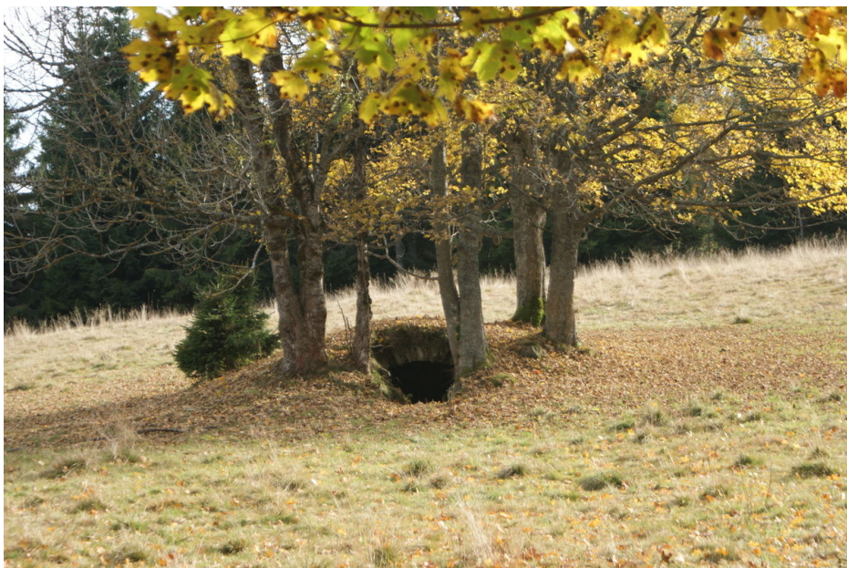
Destroyed cellar across from the house Nr. 35 (G in the map).
