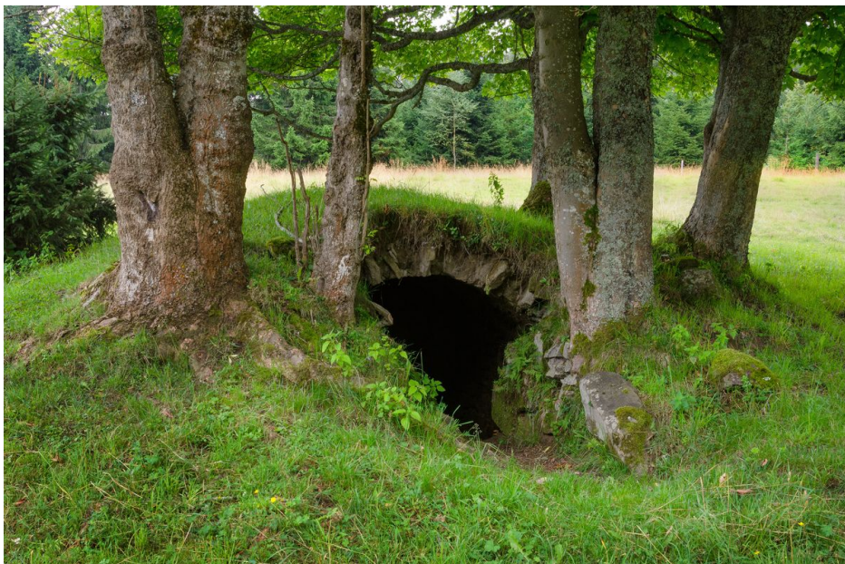
Destroyed cellar across from the house Nr. 35.
