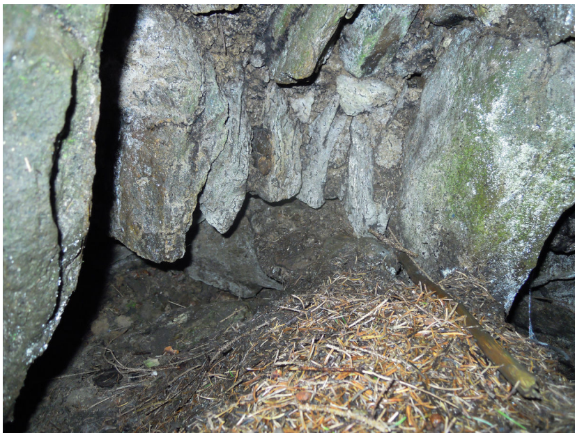
Collapsed vault of a cellar beneath the oven in the western residential wing.
