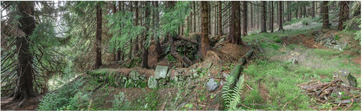
Preserved masonry of the Kotelská shelter.
