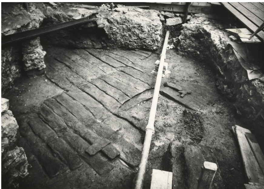
Road paved with wood from the 10th century found beneath the III Courtyard. Prague Castle Archives, 1927.
