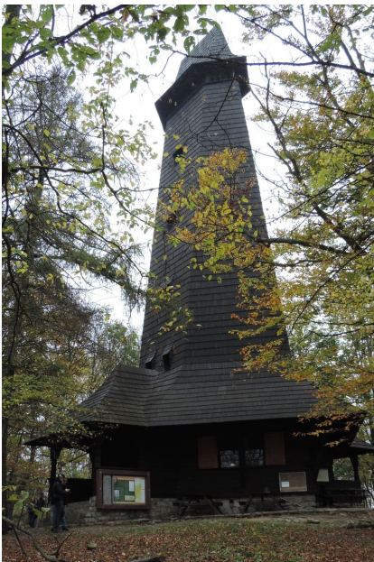
Observation tower at the top of Velký Blaník hill.
