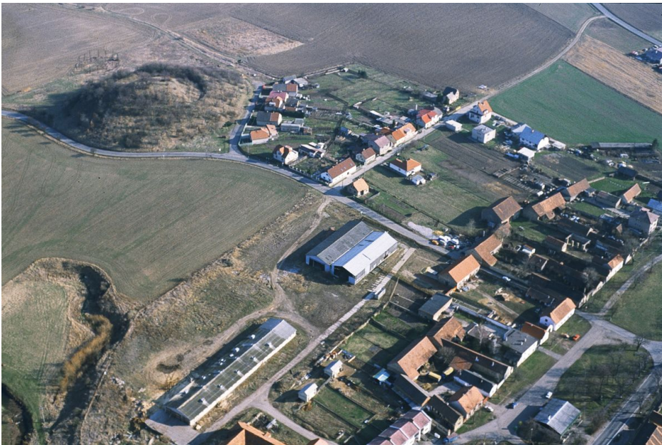
Aerial view of the site, taken from northwest.
