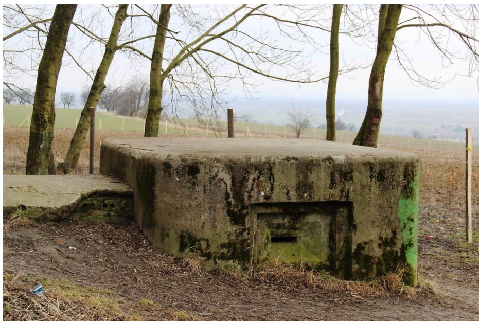
Detail of the embrasure of the concrete bunker near the altitude of the Švédské šance ('Swedish Sconce'). Photo Z. Schenk.
