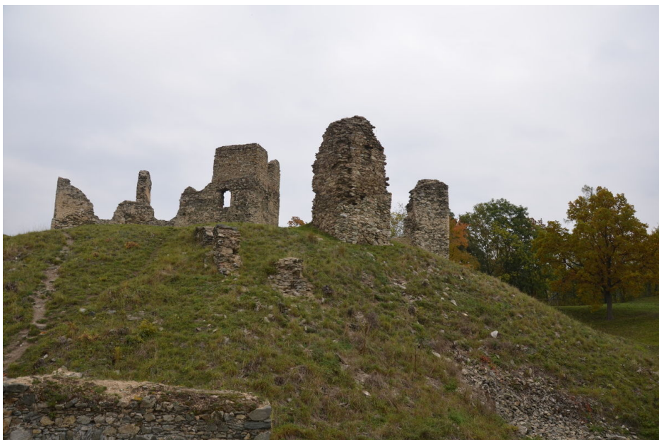
View of the upper ward from the south-west.
