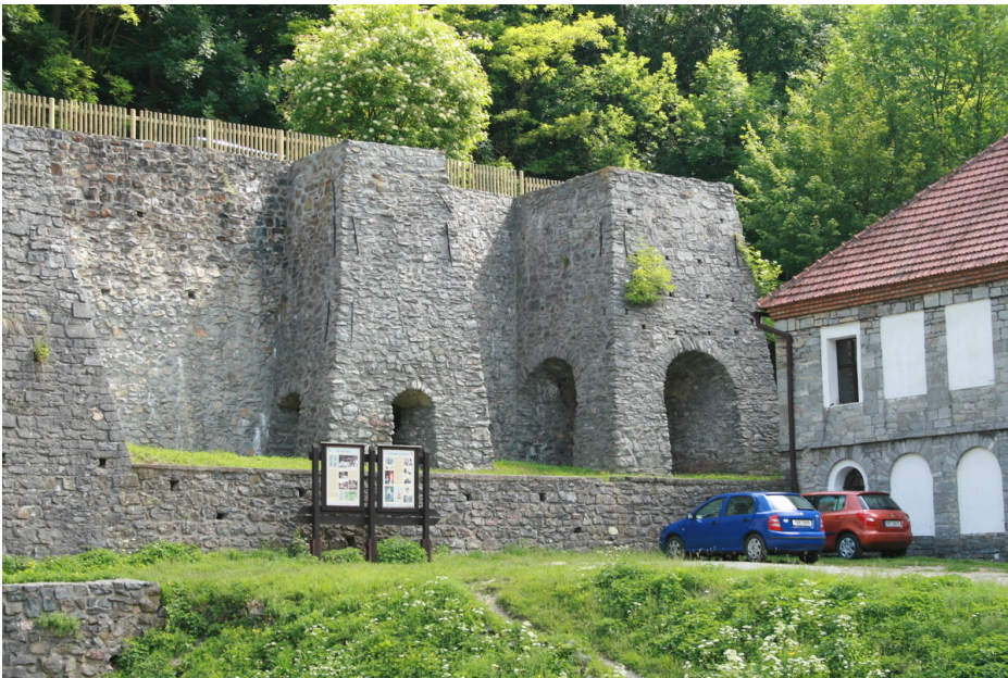
View of the backfill ramp, a pair of lime kilns and the administrative building. Photo K. Sklenář, 2009.
